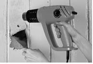
• Using a heat gun at temperatures greater than 1100°F.
